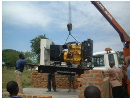
Left: Placing new generator on slab of future generator house (July)
